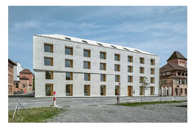
Figure 2: Robust façade with substantial energy-absorbing mass (Baumschalger Eberle Architects Zürich, 2019)
