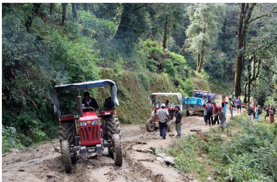
Tractors on the access road to the Arun 3 hydropower plant near Num, Nepal.
