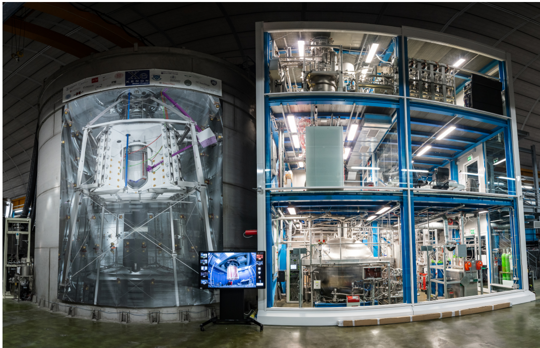
Figure 2.7.: XENON water tank and service building in Hall B of LNGS. The canvas print hung on the front of the water tank depicts a rendering of the inside, where the muon veto, neutron veto, calibration, and TPC structures are shown. The rooms in the service building are used as follows: upper left – cryogenics, gaseous xenon (GXe) purification, gas xenon pumping; upper right – radon distillation column; centre left – DAQ and power supplies; centre right – office space, top part of the krypton distillation column; bottom left – ReStoX1, LXe purification; bottom right – bottom part of the krypton distillation column, GXe bottles. Picture by H. Schulze/XENON Collaboration.
